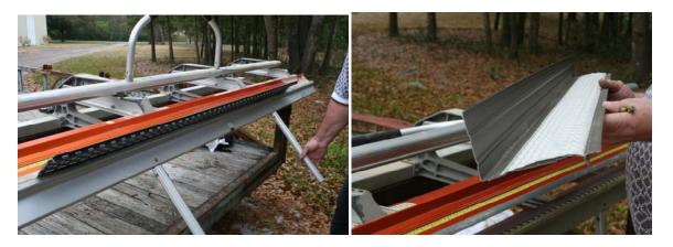
Field forming for fascia mount applications using a small sheet metal hand brake
