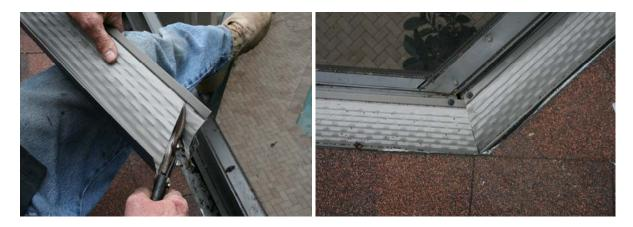
Panels may be easily cut-to-fit using sheet metal snips
